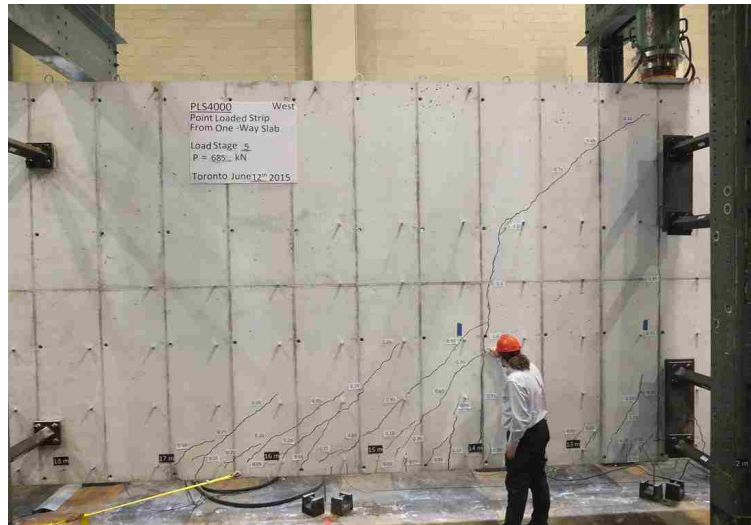
Figure 6.13 – Close-up of shear crack in west side of Toronto beam for phase I
