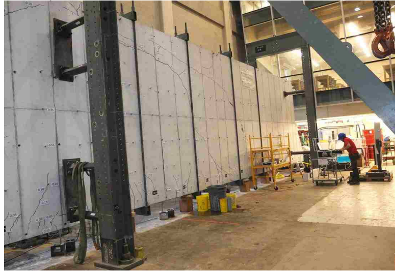
Figure 6.14 – Dywidag bars applied to Toronto beam in phase II
